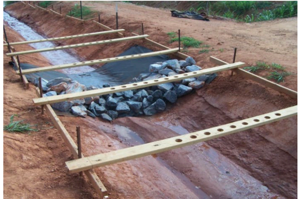
ASTM 7208 ROCK CHECK DAM
